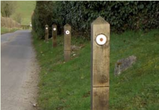
1 Choose appropriate materials. Timber bollards, marker posts and other roadside furniture should be used as they are more in keeping with the rural scene. Generally avoid plastic roadside furniture.
